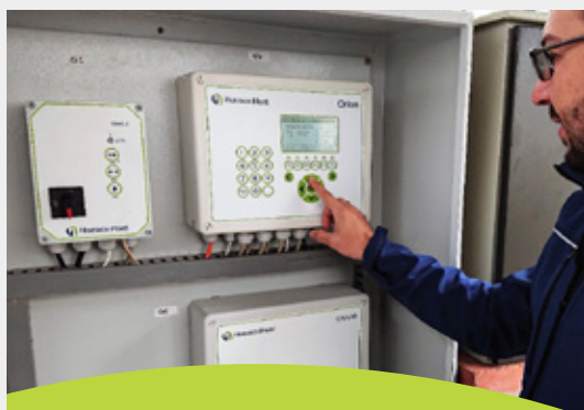
Climate and irrigation computer
